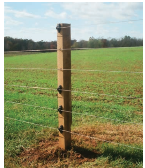
LEFT: Installing black locust fence posts. A chainsaw can be used to make points for easier installation in hard ground. Unlike working with CCA treated wood, littering the land locust wood shavings will not contaminate the soil. RIGHT: Black locust fence post.
