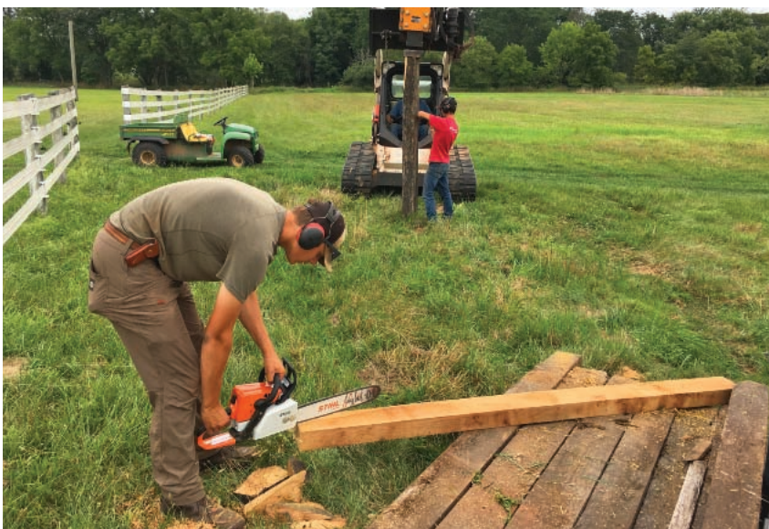
LEFT: Installing black locust fence posts. A chainsaw can be used to make points for easier installation in hard ground. Unlike working with CCA treated wood, littering the land locust wood shavings will not contaminate the soil. RIGHT: Black locust fence post.
